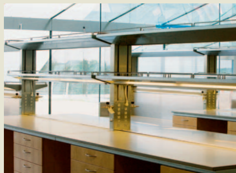
Flexible workspaces: Specially designed bollards enable lab benches to easily take on different functions.
